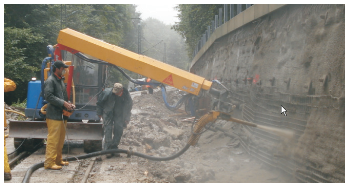
Picture on the left: Mounting of the AL-302.1 onto a Putzmeister carrier
