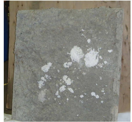
Fig.1 Shotcrete surface prior to application of MULTI-white®
