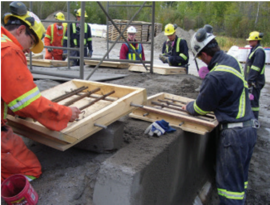
Preparing the Test Panels for Shotcrete Spraying
