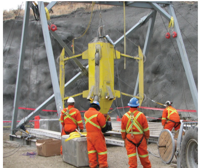
Figure 2: Raise Ranger® completing top meter of 3.5m x 300m deep raise.
