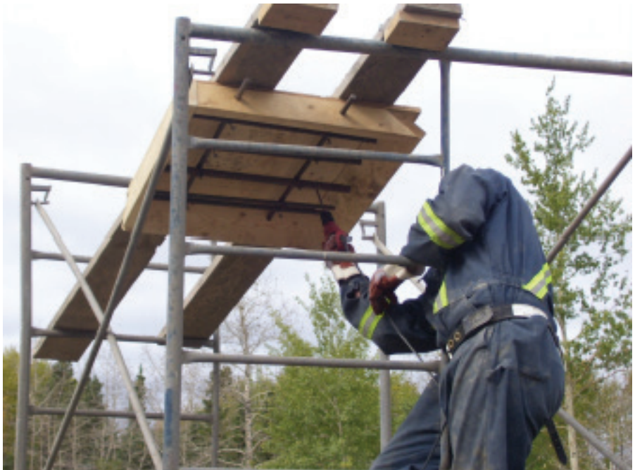
Preparing a Test Panel for Overhead Shotcrete Spraying
