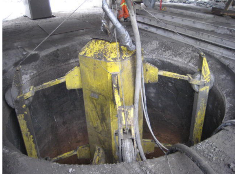
Figure 1: Multicrete Raise Robot™ at top of Raise Shaft
