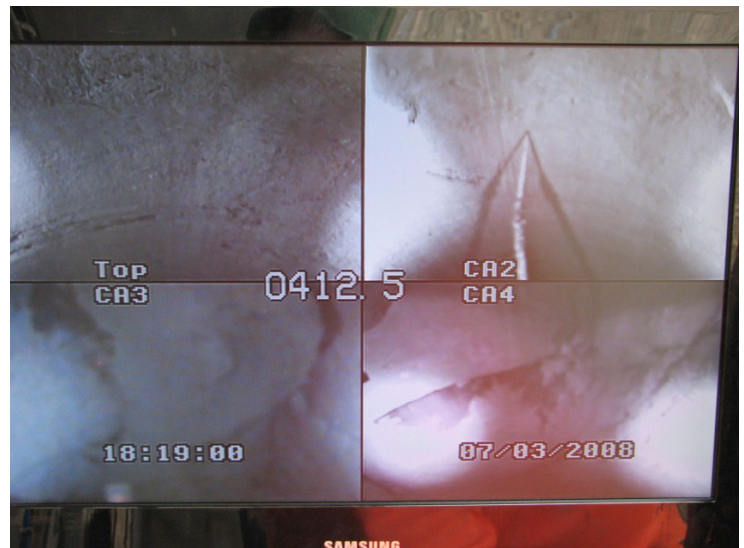
Figure 5: Split screen viewing of shotcrete application
