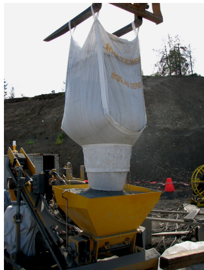
Figure 4: Bags of dry pre-blended shotcrete suspended over pre-dampener hopper
