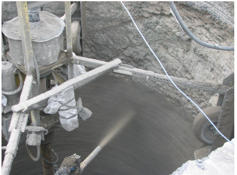
Figure 2: Multicrete Raise Robot™ completing top metre of 3.5m x 300m deep raise.
