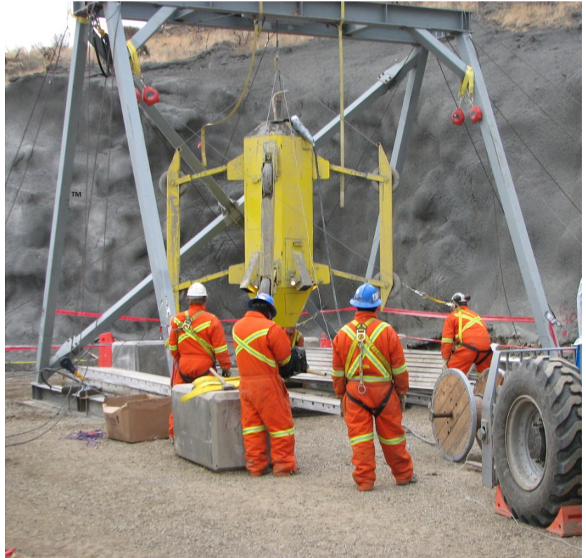
Figure 3: Setting up the Multicrete Raise Robot ™ over the vent raise.
