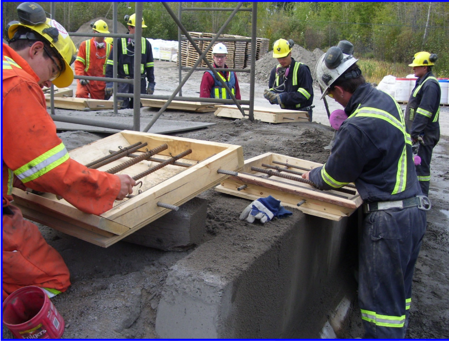
Preparing the Test Panels for Shotcrete Spraying
