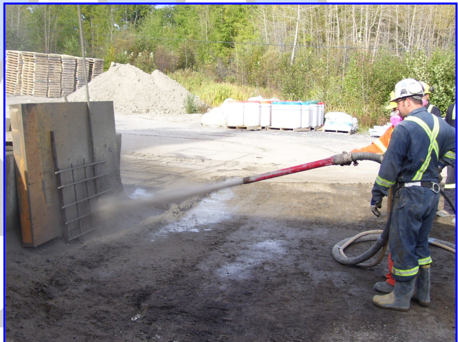
Practicing Shooting Shotcrete Ensuring the Encapsulation of the Rebar
