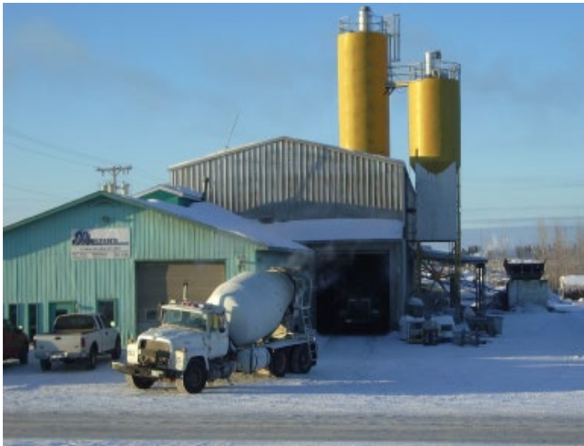
Batch & Redi-Mix Plant Thompson, Manitoba
