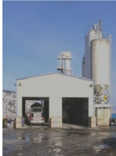
Afton Batch Plant, Kamloops, BC New Gold Mine
